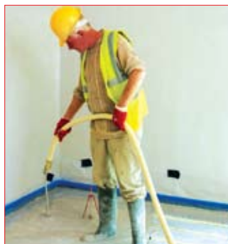
The specialist contractor places the screed and tamps the floor to its final level
