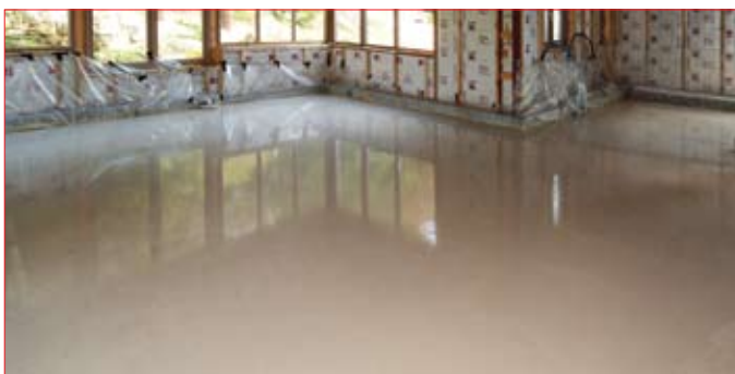
Completed floor after placement
