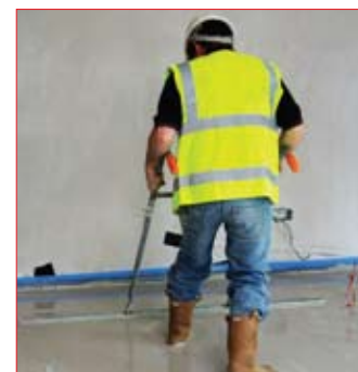
The specialist contractor places the screed and tamps the floor to its final level
