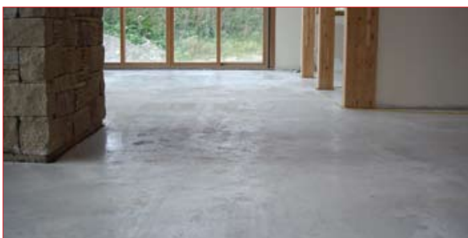
Finished floor ready for handover
