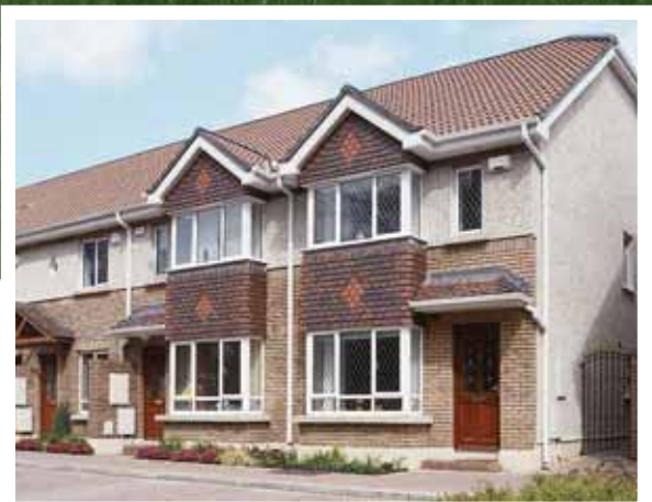
Ashtown Residential Development, Co. Dublin
